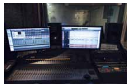
One of the new audio post suites at New York City's Outpost Digital, featuring gear sourced through GC Pro.
