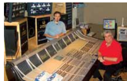
Turner Studios' Erinn Thorpe (left; senior production engineer) and Rick Perry (studio audio manager) with the facility's new mc 2 90 production console
